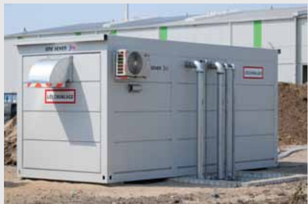
fire fighting system-container
