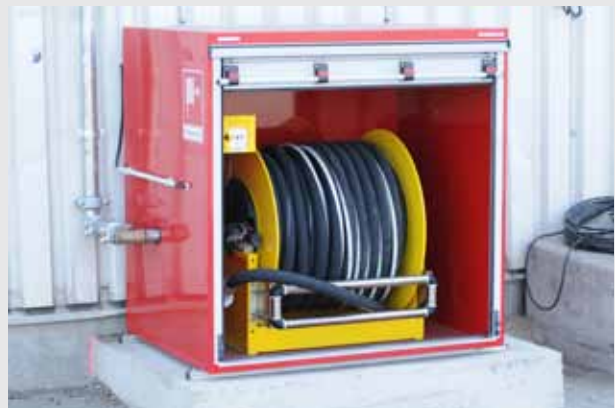
wall hydrant with One Seven® compressed air foam
