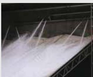
Protection of conveyor belts with nozzles
